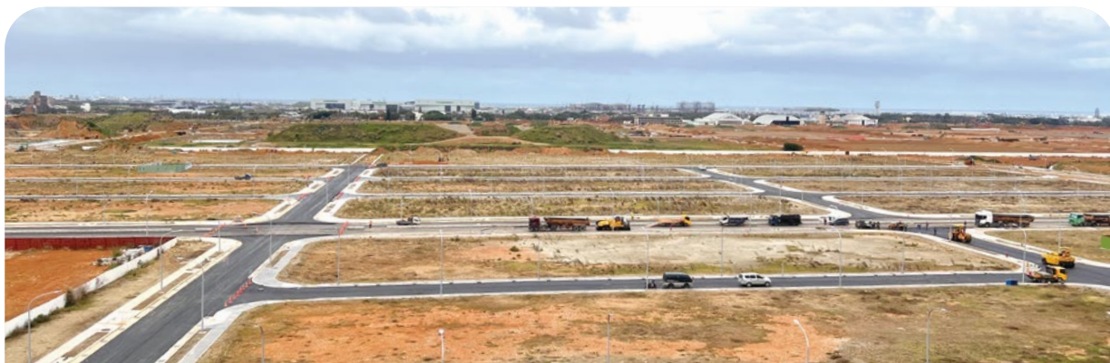
桃園航空城安置街廓 Taoyuan Aerotropolis Project resettlement block engineering
