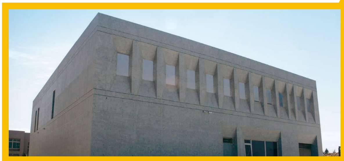
馬公機場助航燈光動力機房 Generator room for navigational lighting aids in Magong Airport
