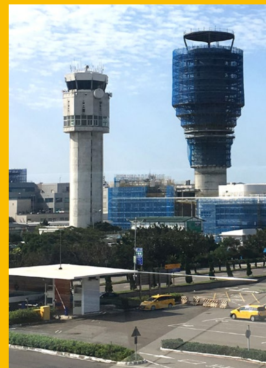
新建塔臺及現有塔臺 New tower and existing tower
