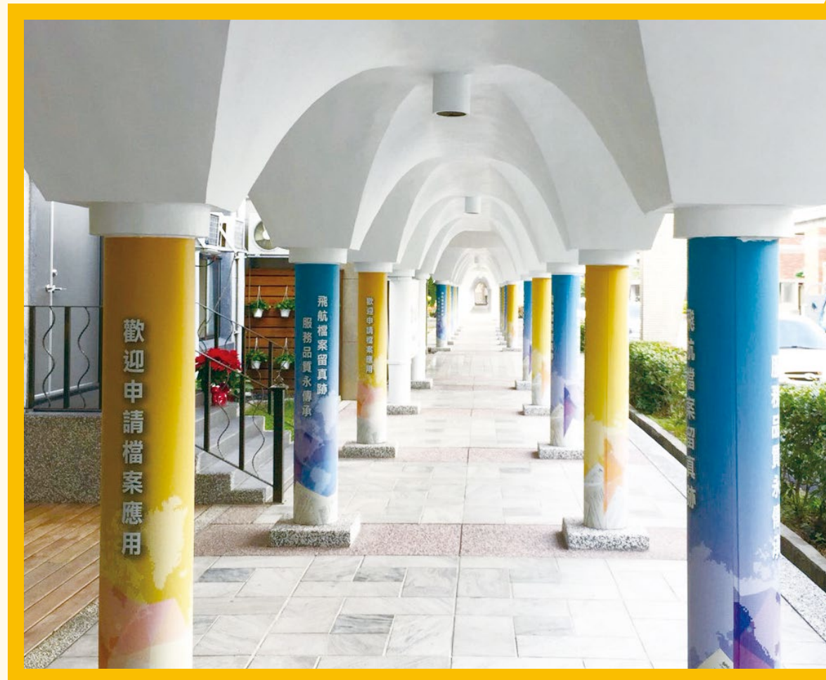
濱江地區油漆粉刷及壁癌處理工程 Painting and Wall mold removal Operation in Binjiang area
